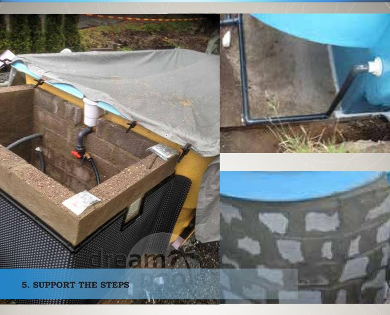
The steps should be supported with concrete blocks, properly checked for the correctness of their level. The fissure between the steps and concrete blocks should be filled with soft foam or it should be salienated all around. On the performed base plate we put the pool and make final checks on the level and the settings. After that we install the water system.
