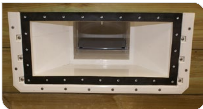
Figure 35 – 1st self adhesive flange
