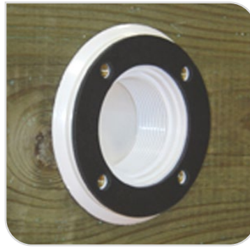
Figure 37 – Applying the gasket
