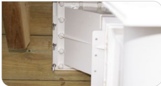
Figure 34 – fasten the skimmer in position
