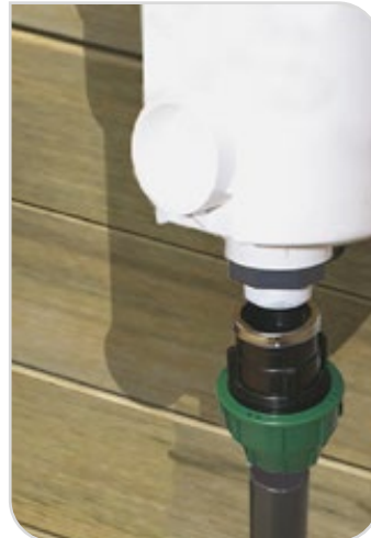
Figure 43 – Rigid descending pipe
