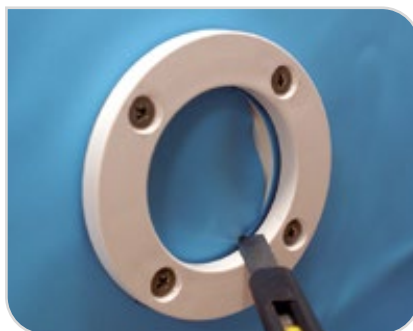
Figure 53 – Cut out the liner
