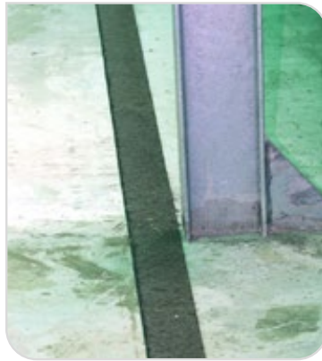
Figure 15 – unrolling the asphalt strips
